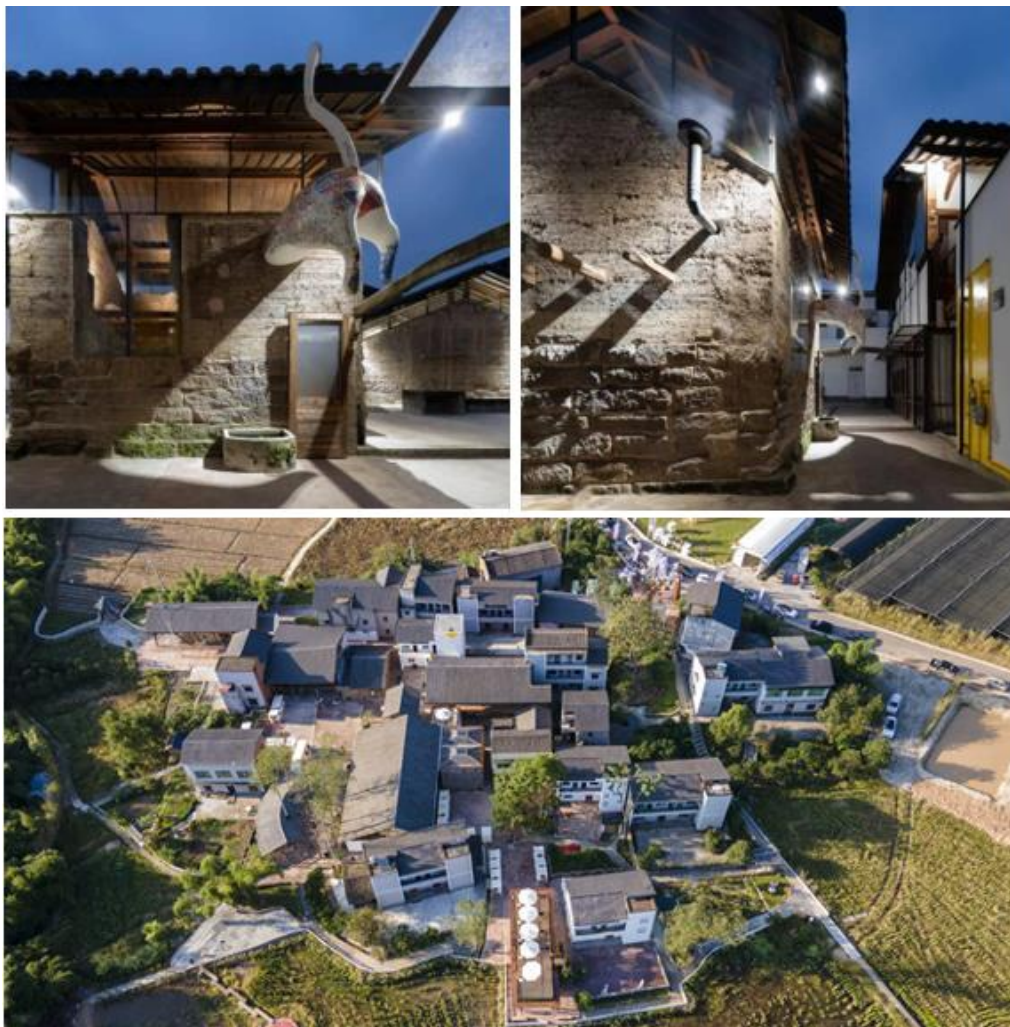
Figure 2. Appearance of Jangjun Villager Residence after restoration (Photo source taken by the author)
