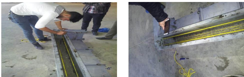
Plate 1. Steel mold used and concrete casting process
