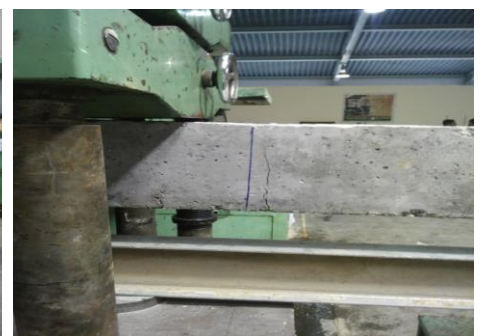
Plate 3. Beam flexural cracks
