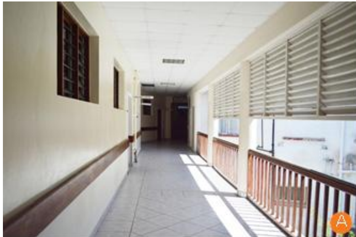
Figure 4. Reviewing sustainable site planning with natural lightning.
