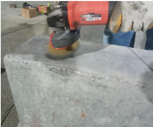
Figure 2. Beam soffit preparation before CFRP sheets installing
