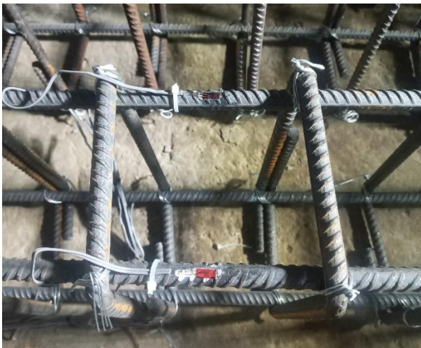
Figure 4. Strain gauges installed on the tensile reinforcement
