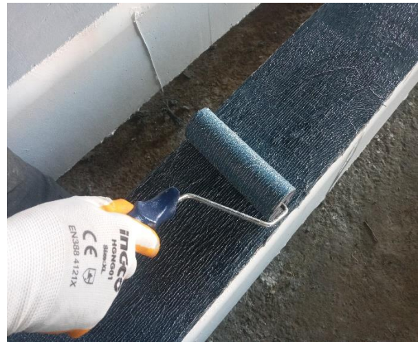
Figure 3. Adhering (CFRP) sheets
