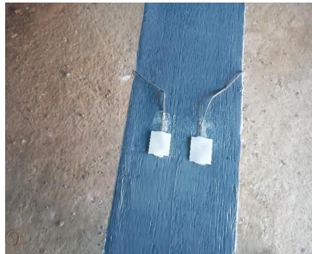
Figure 5. Strain gauges installed on (CFRP) sheets
