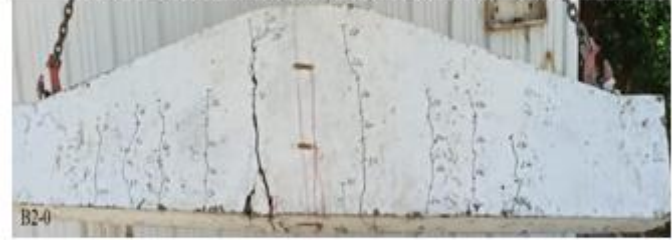
Plate 8. The failure of the (B2-0) beam
