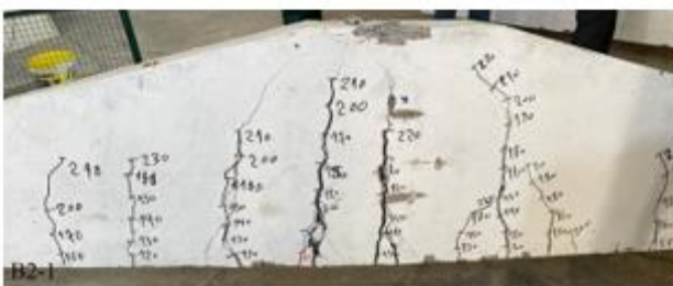
Plate 9. The failure of the (B2-1) beam
