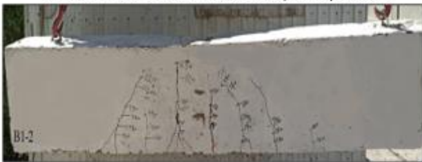
Plate 3. The failure of the (B1-2) beam
