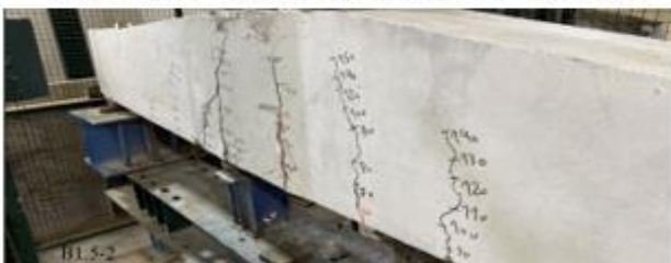
Plate 7. The failure of the (B1.5-2) beam
