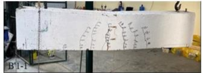
Plate 2. The failure of the (B'1-1) beam
