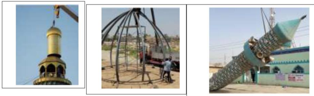
Figure 5. Transformation of the body of the minaret from a building to a shell made of metal only
