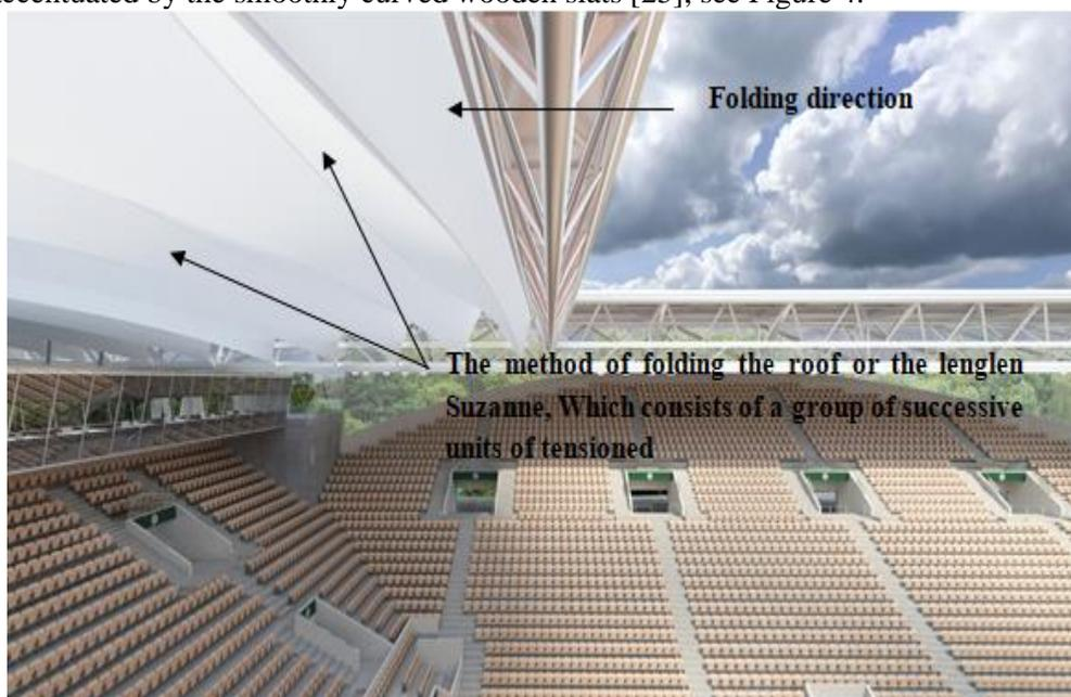
Figure 1. The roof of the Lenglen tennis court in France shows how the folding roof opens and closes [28]
