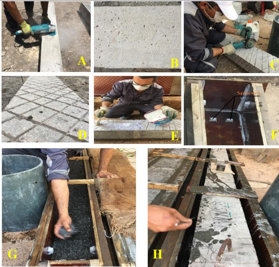
Figure 7. The procedure of strengthening fire damaged LWC beam specimens
