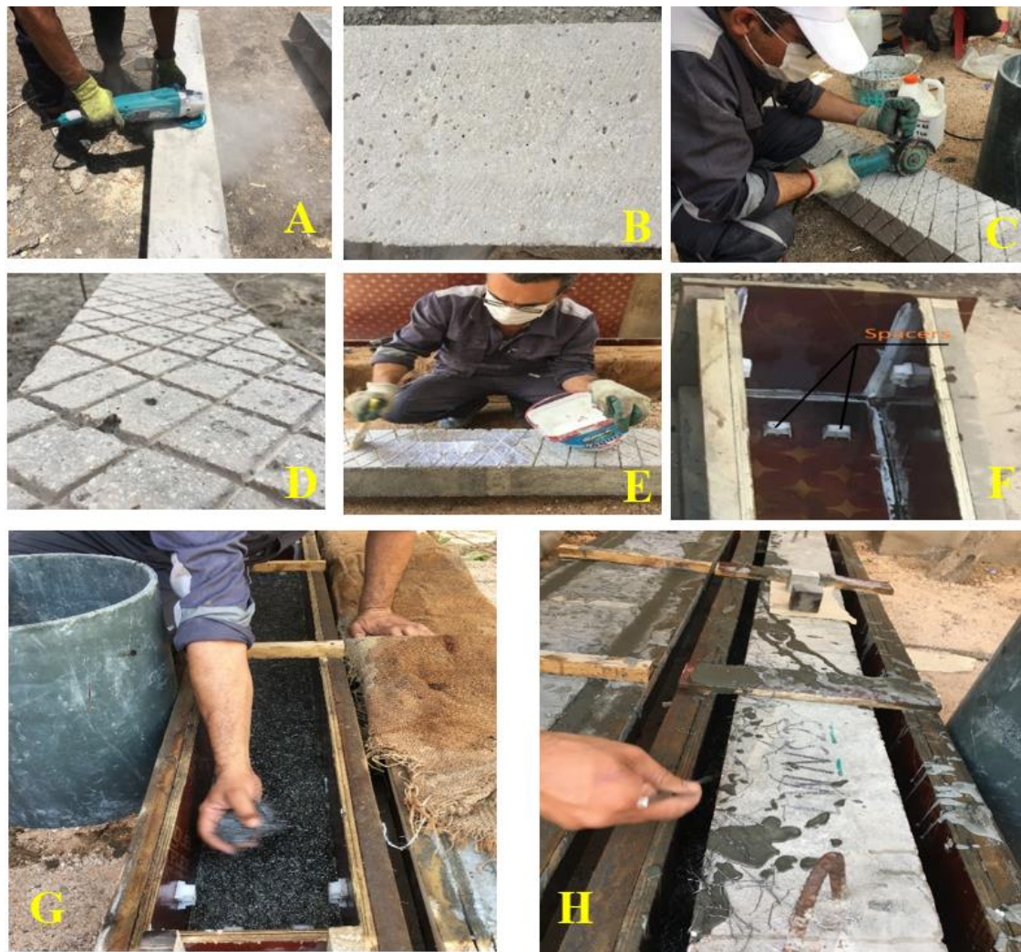
Figure 9. Process of strengthening the fire damaged LWC beam specimens
