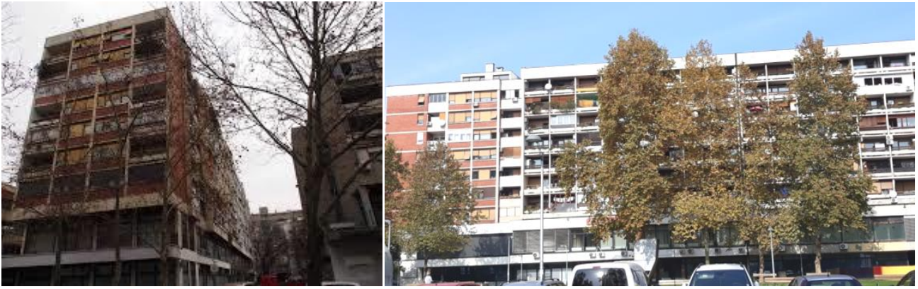
Figures 10 and 11. Residential building in Ivan Visina Street, Siget, Zagreb. Source: Adapted from [8]
