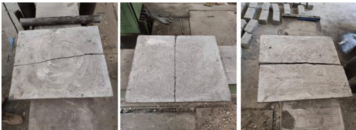
Figure 7. Cracking pattern of simply supported ECC concrete
