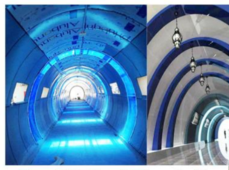
Figure 12. The internal lighting units of the bridge (researchers)
