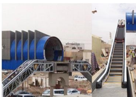
Figure 13. The bridge structure and its connection point with the escalator (researchers)
