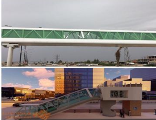
Figure 9. Smooth concrete columns that are not compatible with the proportions of the bridge and are devoid of details and decoration (The Researchers)
