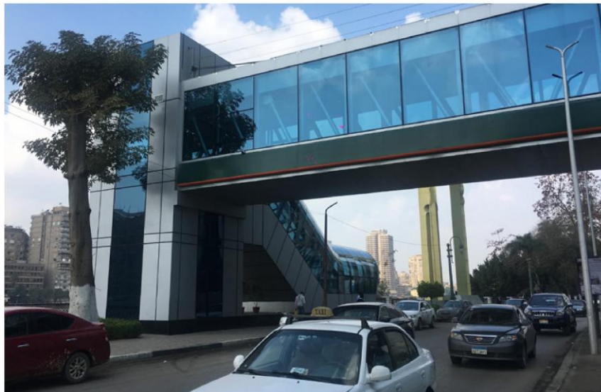
Figure 2. Shows the visual aspects of the pedestrian bridge
