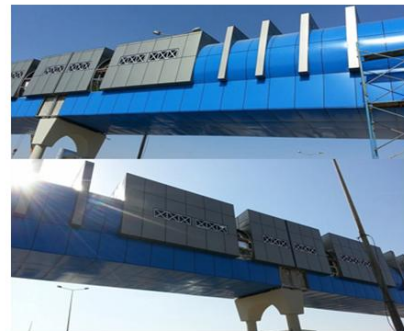
Figure (10) The mass formation of the bridge, the lack of color coordination, and the use of the alcobone as a sheathing for the bridge (researchers)
