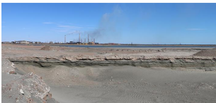
Figure 1. Tailings pond of Balkhash enrichment plant
