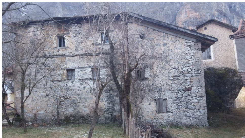
Figure 9. Adaptation of the house by addition of new cross wing on the house in hamlet Cosici
