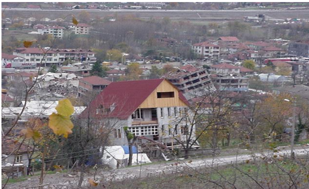
Figure 2. Destruction in Merkez District, Kaynaşlı, after the 12 November 1999 earthquake [14]
