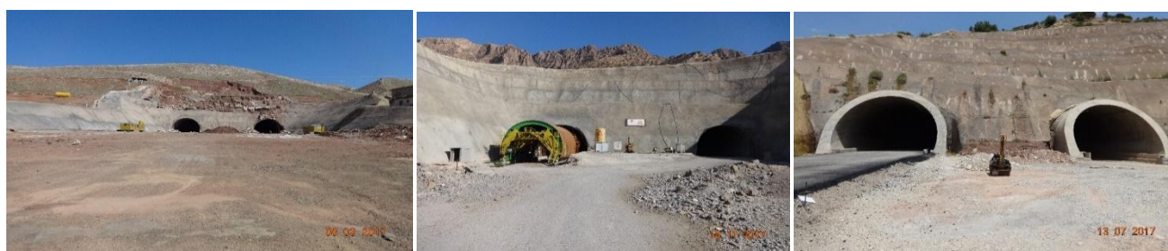
Figure 2. Haybat Sultan, Bani harrier and Salahuddin (Permam) Tunnels /located area of study
