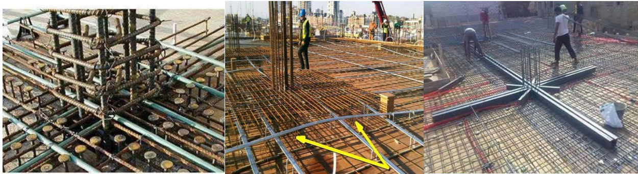
Figure 2. Punching shear preventers
